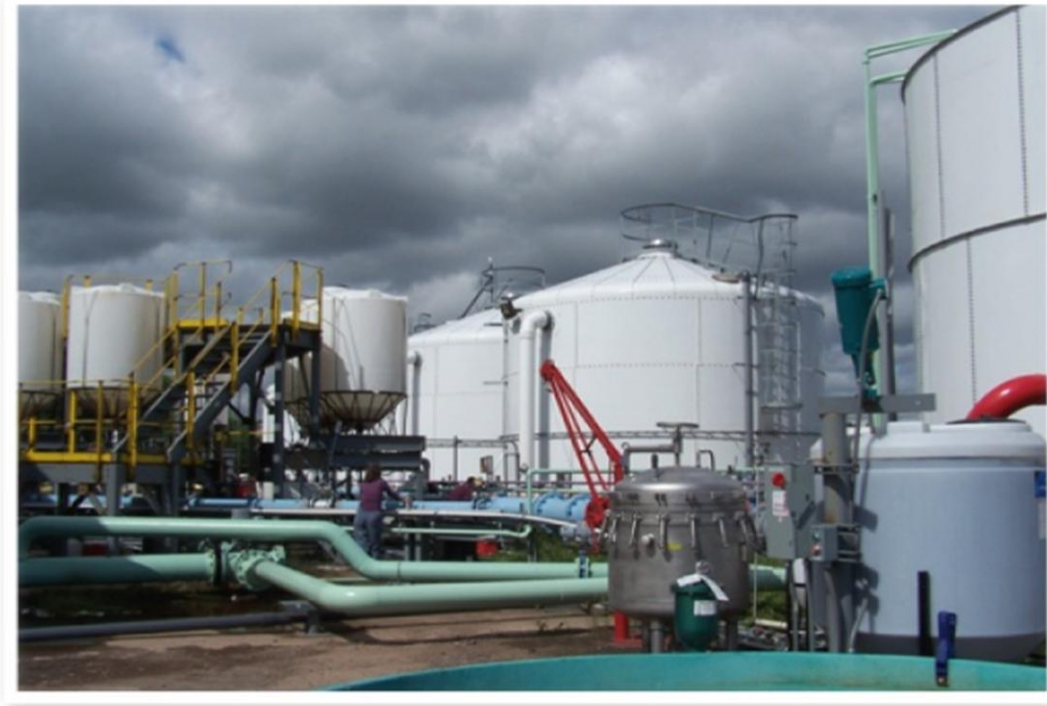
Figure 3. Photo of the GSI Land-Based RDTE Facility.
